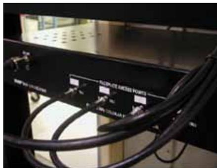
**The CDS system uses the same coaxial cable as used for cable television and may be easily implemented over previously installed cabling.**
